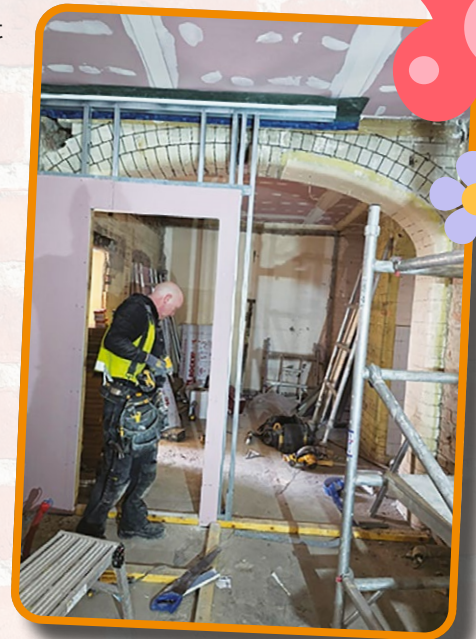
Conversion works taking shape at the former Police Station building.
